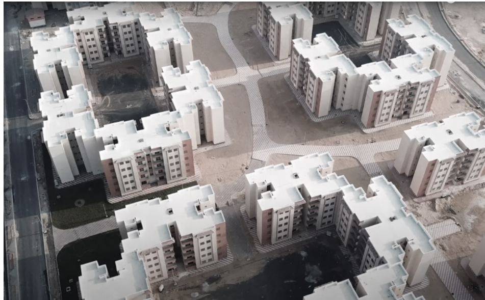
Figure 25 Open Spaces in the Social Housing Units. Source: NUCA
