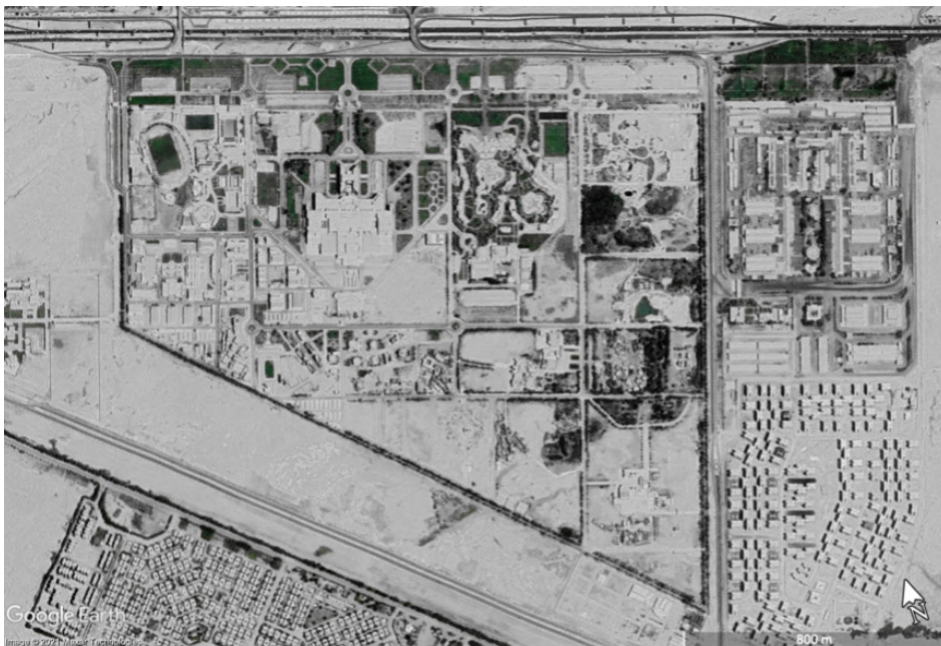
Figure 16 The Media City in the 6th of October City. Source: Google Earth
