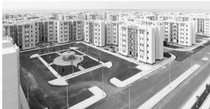
Figure 13 Urban Segregation in the city. Source: NUCA
