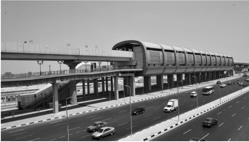
Figure 24 One of the completed monorail stations. Source: www.tahiamasr.com/612759 .
