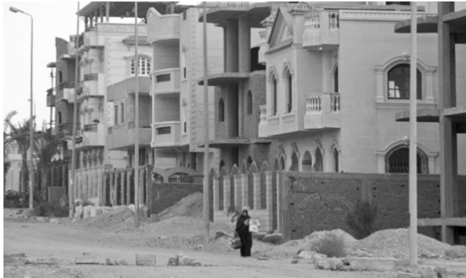
Figure 43 Private Housing built by individuals in New Cairo. Source: Sean Smith for the Guardian
