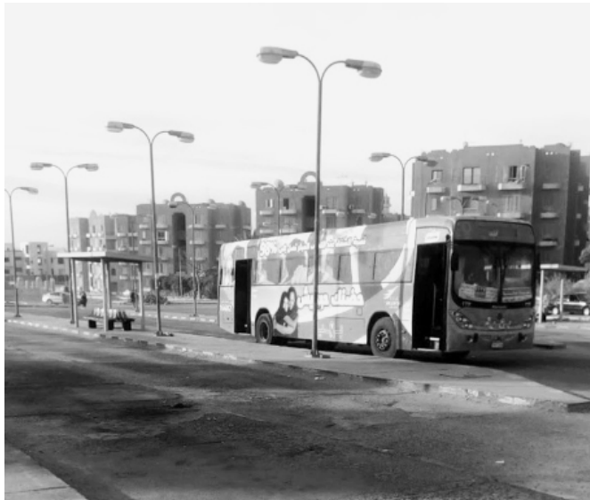
Figure 8 Deserted Bus Terminal in New Cairo City, Third Settlement Terminal. Photo by: Abdelrahman Nagi, Google Maps
