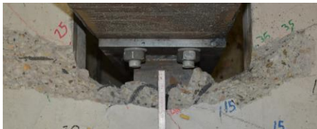
Figure 14 Concrete crushing in the area of connection after the end of experiment No.10. Placement of first shear stud close to face of column \rightarrow more intensive concrete cracking and crushing (at concrete cover).
