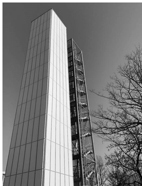
Figure 1. High-rise demonstrator with adaptive load-bearing structure (l) and access tower (r) at the University of Stuttgart. Source: Institute for Lightweight Structures and Conceptual Design (ILEK).
