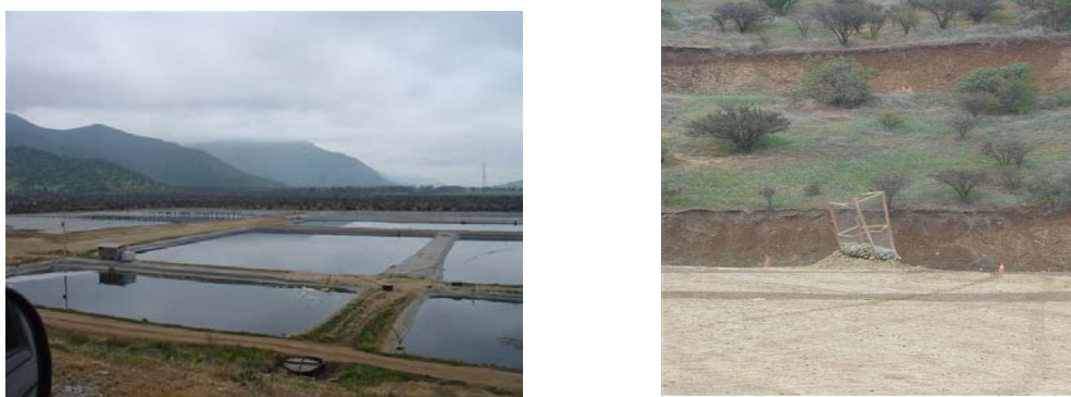
a) b) Figure 4.7 Landfill Santiago Poniente (background research 2007) a) Leachate pools b) Biogas collection
