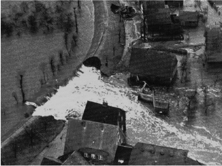
Figure 1.1: Water flows through a broken dike
