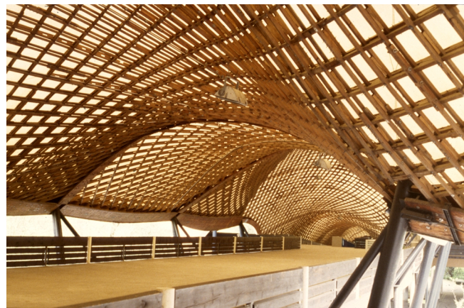
Mannheim, Multihalle: Passage-way connecting the two shells
