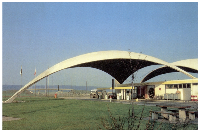
Concrete shell roof of the gasoline station at Deitingen, Switzerland (Heinz Isler)
