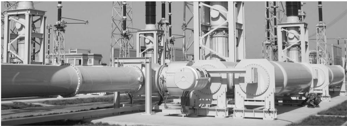
Figure 1: Pictures of 'Jingmen' 1100 kV substation
