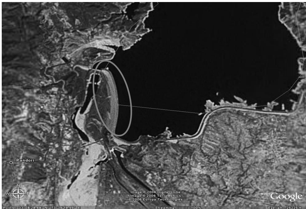
Figure 3.1: Top view of Mangla dam (by Google earth)
