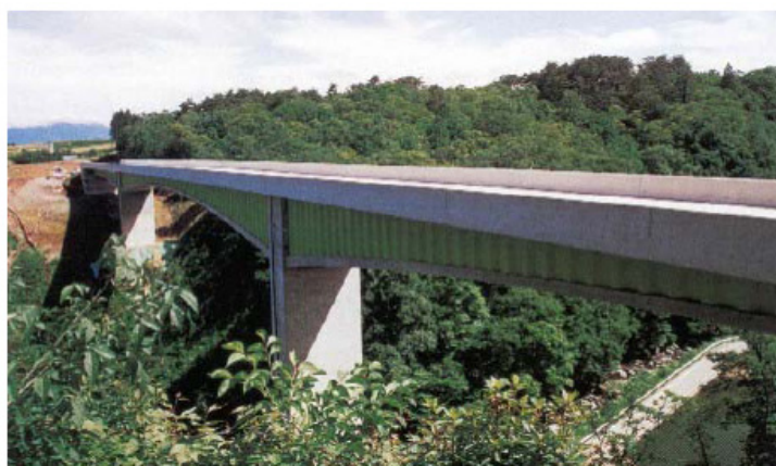
Abb. 2.18: Hondani-Brücke [VITEK, V. (2003)]
