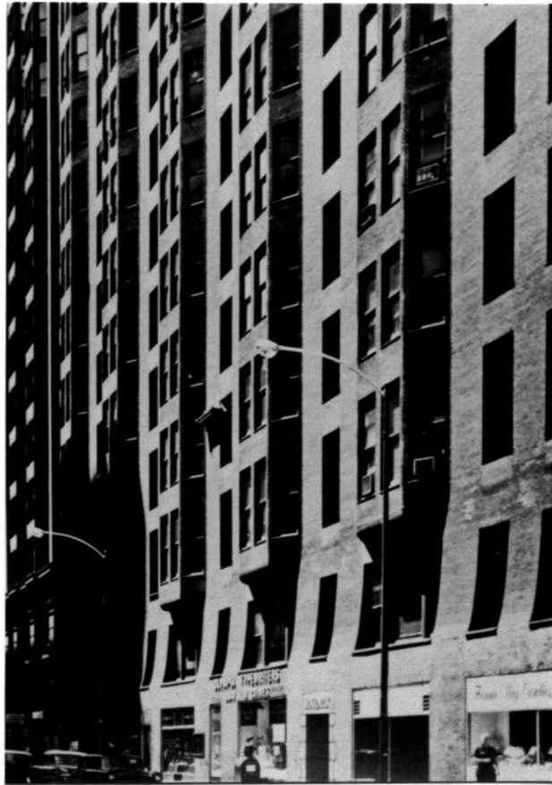
Chicago, Monadnock Building 1891
