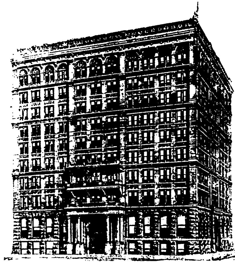
Home Insurance Building, Chicago, Ill., 1884-85 William Le Baron Jenney, architect. This celebrated building came closest to being the first true skyscraper, with fully developed skeletal construction.
