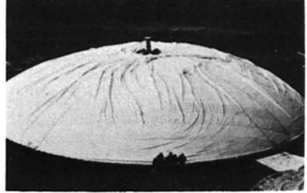
Fig.9: Rainwater interceptor tank: Inflated formwork.
