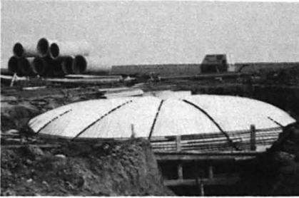
Fig.9: Rainwater interceptor tank: Inflated formwork.
