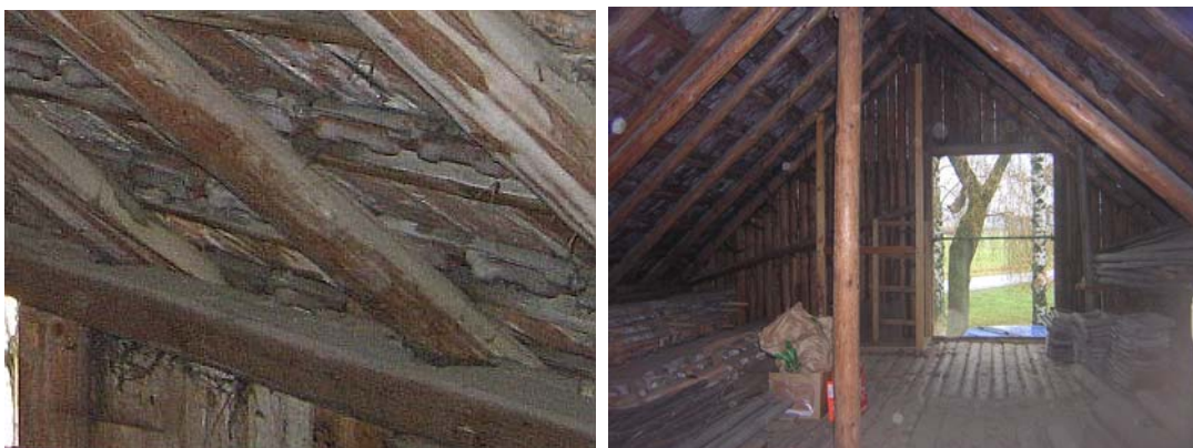
(a) Clamping at the support due to a large groove depth for the connection between rafter and purlin (b) Load transfer to the end wall by means of the battens
