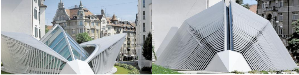
Figure 18- Transformable roof of Emergency Center by Santiago Calatrava (Calatrava 2009)
