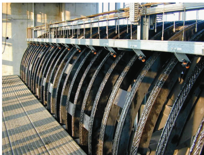
Figure 1: Sheaves of a ship lift
