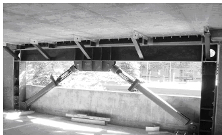
[Source: www.staaleng.com] b) Viscous dampers
