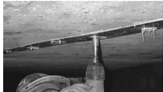
d) Mechanically anchored FRP laminates (Lopez & Nanni, 2006)
