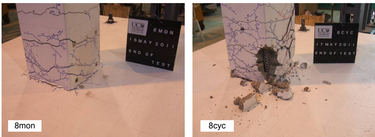
Figure D.16 Monotonic and cyclic test on Specimen 8: Damage pattern after testing
