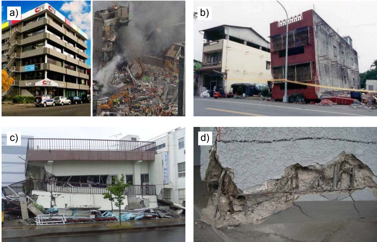
Figure 1.3 Failure of columns: a) CTV building before and after 2011 Christchurch Earthquake (Source: NZ Herald); b) and c) Shop houses after pancaking during 1999 Chi Chi and 2011 Tohoko Earthquakes (Source: EERI, ISE); d) Column-to-foundation connection failure during 2011 Tohoko Earthquake (Source: ISE)
