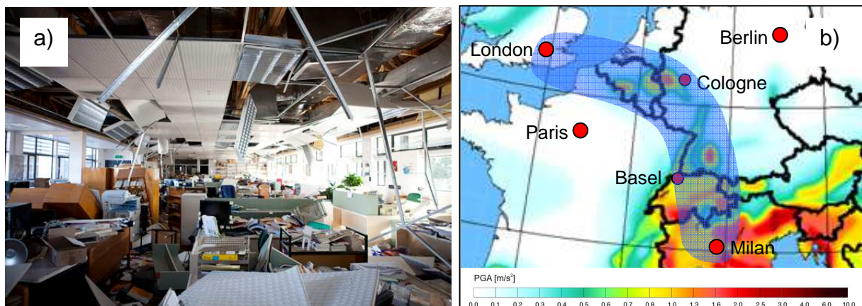
Figure 1.1 a) Collateral damage in office after the Darfield Earthquake 2010 (The Press, Christchurch); b) Seismic risk map of central Europe (after Grünthal, G.; Arvidsson, R. et al. (2004)), and “Blue Banana” indicating high concentration of people and assets (after Brunet, R. (2002))
