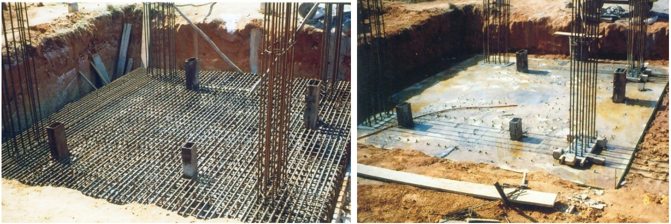
Figure 8.10 Construction of Raft Foundation with Rock Anchors
