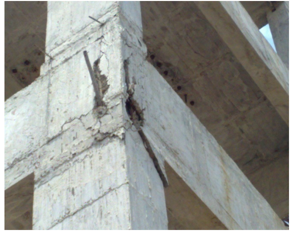
(b) Beam bars bursting out of cover for the joint of CL 19 (2 nd floor)
