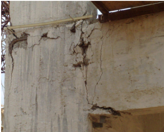
(c) Flexural and bond failure of beam at joint CL16 (1 st Floor)
