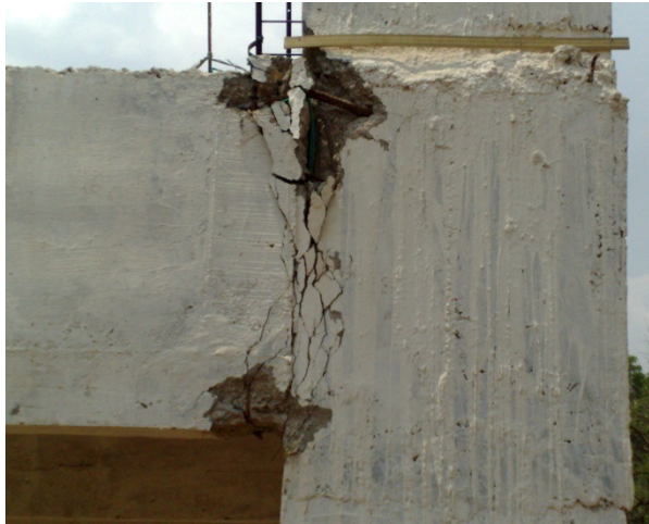
(a) Flexural failure of beam BF 205-1
