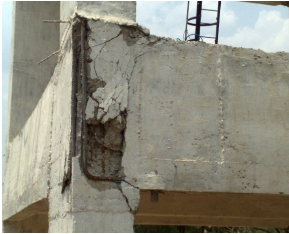
(a) Joint shear failure of CL 19 (1 st floor)
