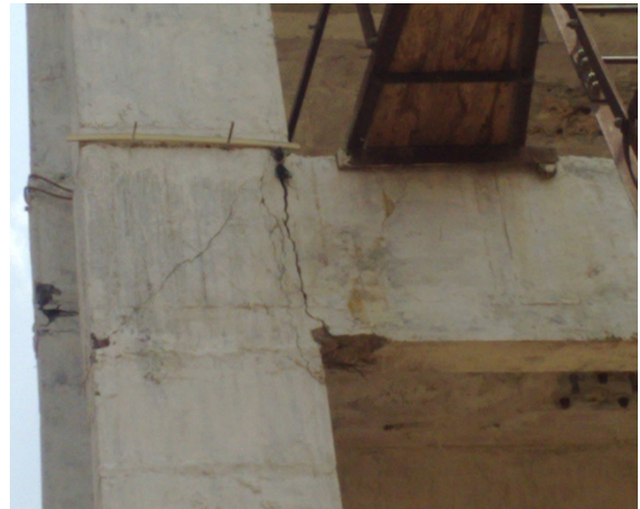
(d) Joint shear cracking and flexural cracking of beam at CL16 (2 nd floor)
