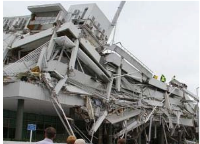
(b) 2011 Christchurch Earthquake
