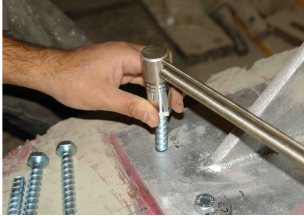
Figure 10.4 Concrete screws used for retrofitting of JT1-5
