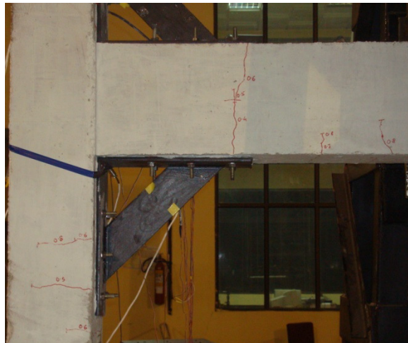
Figure 11.27 Crack patterns observed after the base excitation of 0.8g
