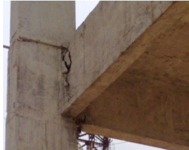
(b) Torsional failure of beam BF223-1
