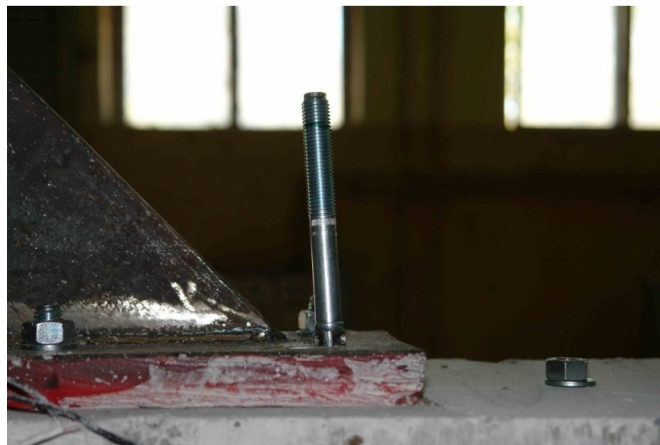
Figure 10.5 Expansion anchors used for retrofitting of JT1-6
