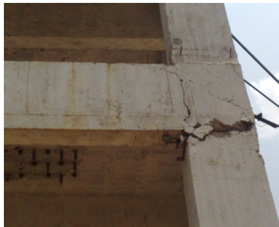
(e) Joint shear, beam-flexure and bond failure of beam bars at CL20 (2 nd floor)
