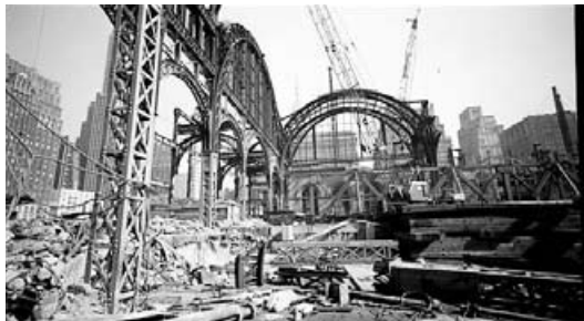
▷ Abb. 3-3: Abriss der Pennsylvania Station (1963)
