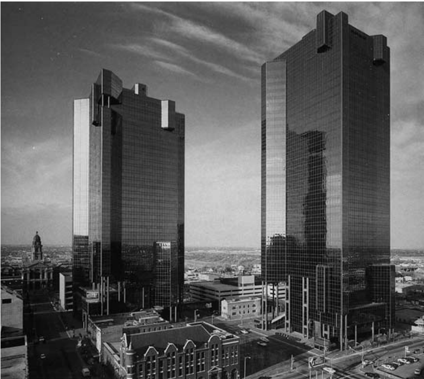
△ Abb. 5-14 und 5-15: Paul Rudolph: City Center, Fort Worth, Texas (1979–83)
