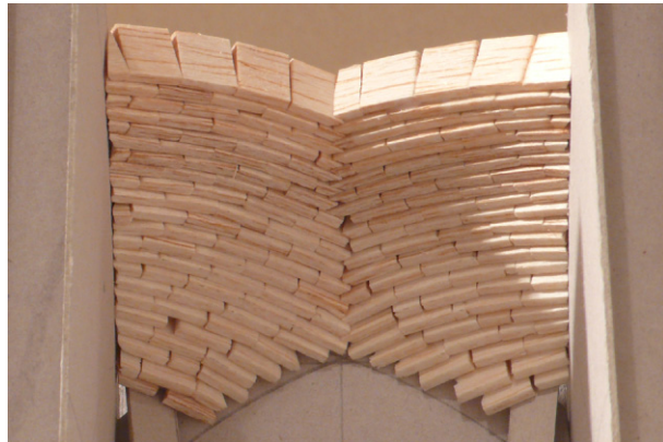
Figure 15 Alternative pattern for the vault masonry, simplifying construction in the earlier phase (author).
