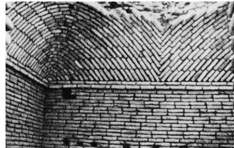
Figure 1 A vault of the "trompe d'angle" type: historical example (Besenval 1984, after Pugachenkova). Note the courses of the masonry, which depart with diagonal inclination, forming arches over the corners of the vault.
