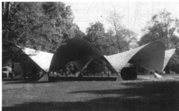
Fig. 4 — Glass fiber reinforced shell, Stuttgart, 1976.
