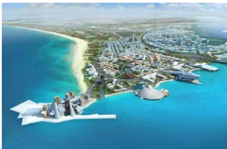
Fig. (6.10) The new Sadiyat Island development, Abu Dhabi shows that the design of the public individual buildings provides a highly defined visual image definition that a coastal city can provide. The buildings enhance orientation, due to the existence of strong and unique identifiable elements.
