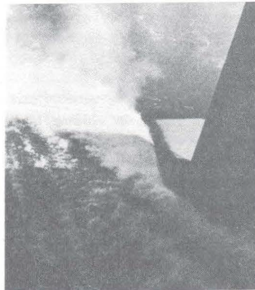
FIG. 1.1 AIR ENTRAINMENT IN FREE SURFACE FLOWS (Aviemore Dam, New Zealand [86] )
