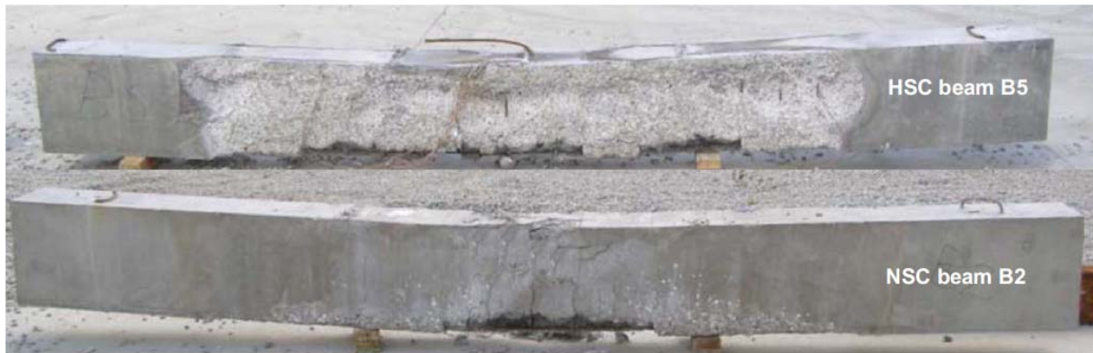
Figure 13 Spalling in NSC and HSC beams under design fire exposure [19]
