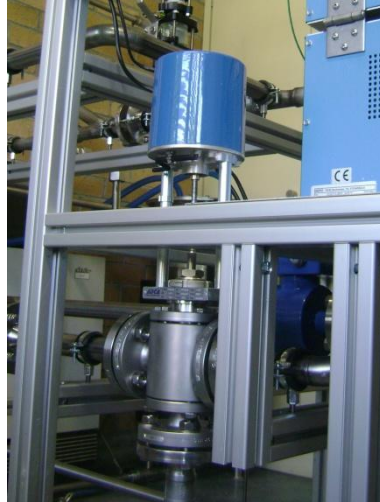
Figure 3-16 The electric actuator and 3 way valve used for the flow control
