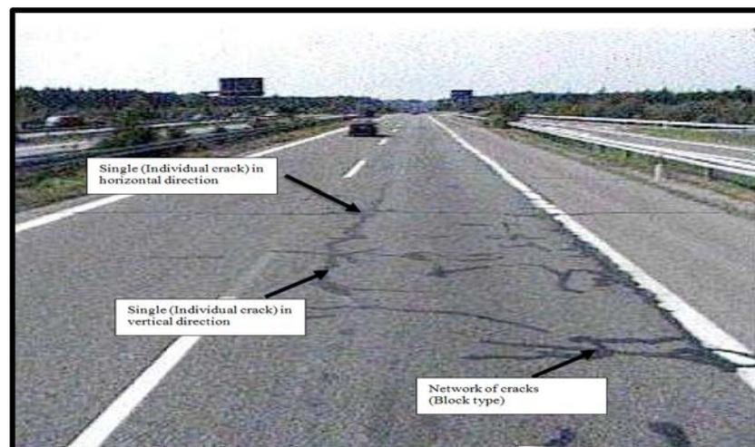
Figure 2.1: Cracking (FGSV 2006).
