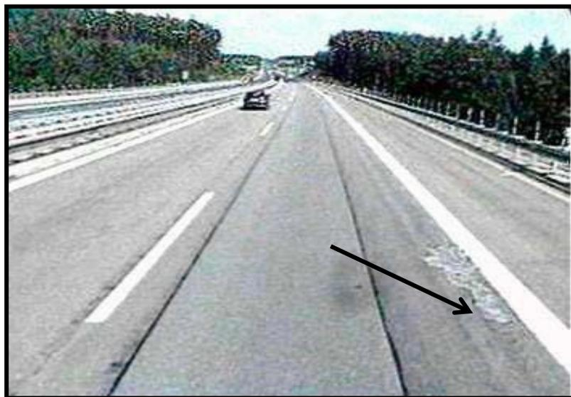
Figure 2.3: Out-breaks (potholes) (FGSV 2006)
