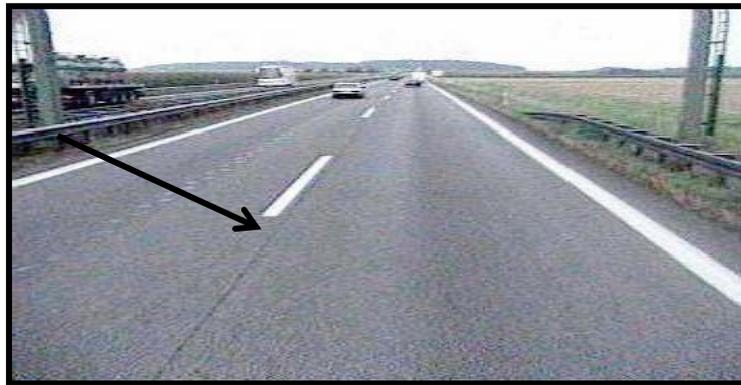
Figure 2.4: Open work seams (FGSV 2006).
