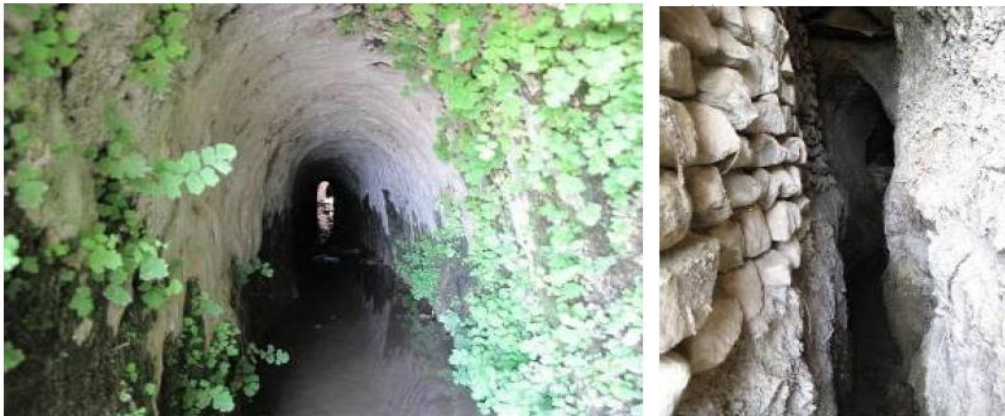
Plate 4.7: Round arch karez tunnel in limestone at Zimzimuk (L); Pitched and pointed arch Sarsula karez at Girdashekhal (in limestone) (R)
