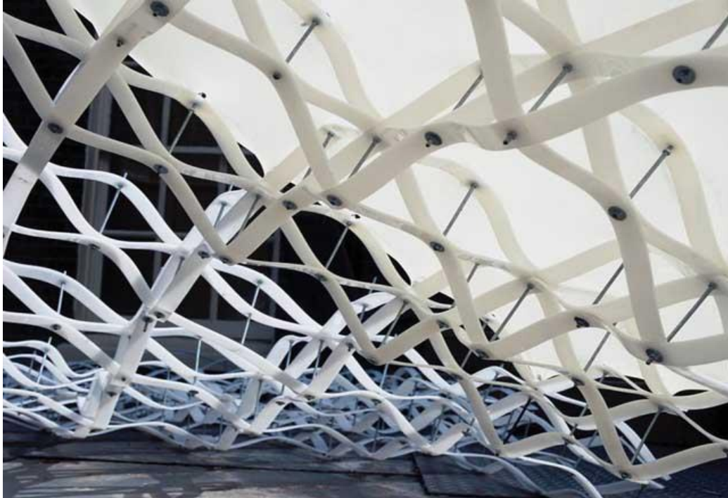
Figure 7.12: A 3D Hybrid structure can generate various surface geometry by controlling the strut lengths between the chords. (Source: http://www.achimmenges.net )
