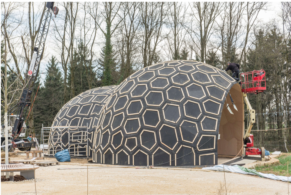
Figure 13.3 Top: Temporary supporting frame work with the section geometry of the inner surface of the plate shell is used here to facilitate the correct positioning of each plate during installation. Bottom: The prefabricated modules of thermal isolation and waterproofing are installed.
