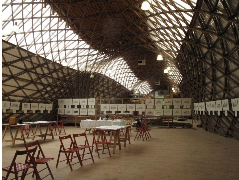
Figure 2.6: Inner view of Downland Gridshell
