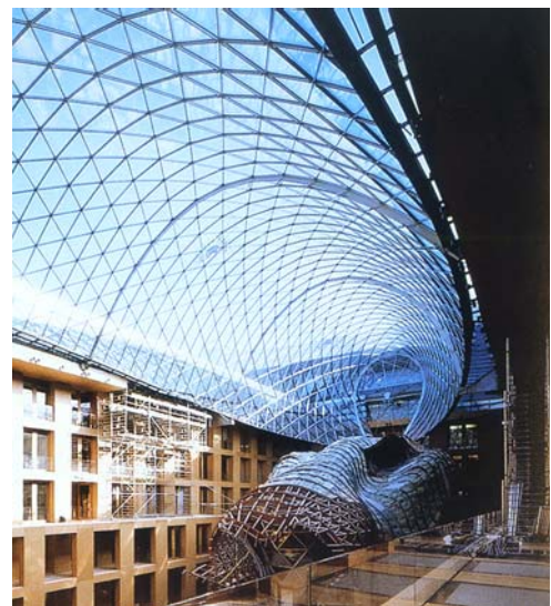
Figure 3.19: View of roof in DZ Bank, Berlin [Schlaich et al 2003]
