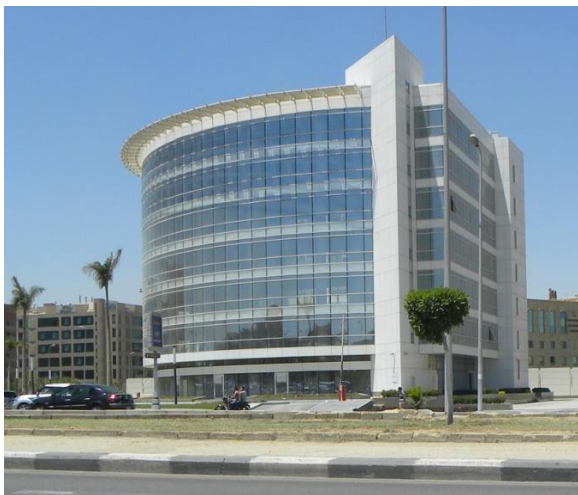
Figure 1 - 3: Unoccupied office building in the fifth settlement, Cairo. The building constructed in 2013 in the Elteseeiny road, with fully and clear glazed facades, exposed to the solar radiation all day without any external solar-protection (By researcher).
