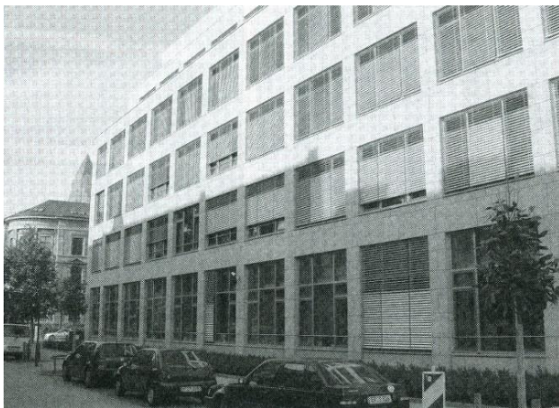
Figure 7 - 25: Venetian blinds divided into two independently functional sections, University of Karlsruhe (Voss, et al., 2007)
