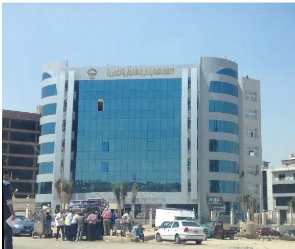
Figure 1 - 8: The general union of the Egyptian commerce chamber building in New Cairo, the building is an administrative governmental office building, constructed in 2013 with highly glazed façade. The southern facade shows no installations of external shading devices to protect it from the extensive solar radiations in Cairo's Hot-arid climate (By researcher).
