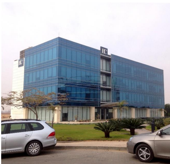
Figure 1 - 4: HC Office building in smart village, near Cairo - Alexandria road. The picture was taken in February with a partially cloudy sky conditions. However, the occupants also pulled down their internal shading for solar protection and ignoring the external green view (By researcher).
