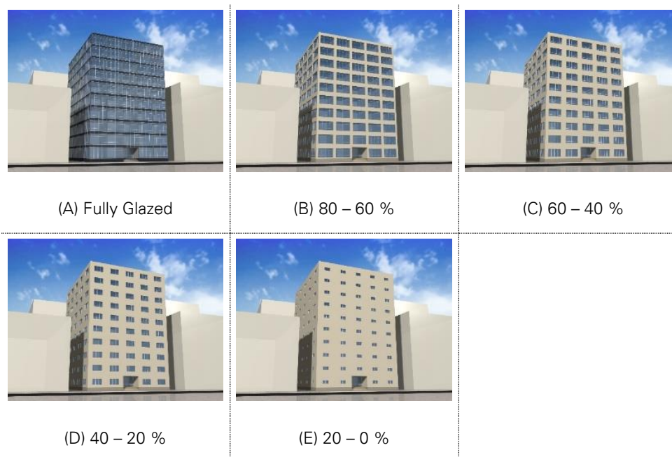
Figure 9 - 42: The given 5 pictures representing different external glazing ratios for an office building in Cairo
