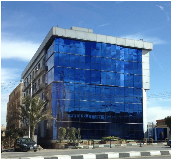
Figure 1 - 6: Office building in El-Mokattam district, Cairo. The street façade of the building is fully glazed with tinted and reflective glazing, but with no external shading devices (By researcher).
