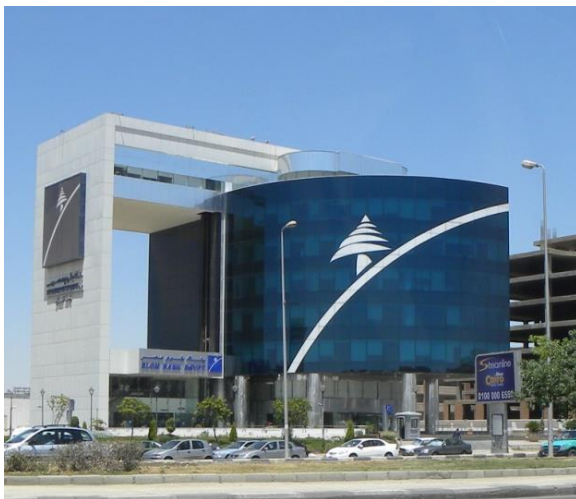
Figure 1 - 1: BLOM Bank building in the fifth settlement, Cairo. The Southern façade of the building is constructed with highly tinted glass. However, this did not prevent the users from pulling down their internal curtains as a protective action towards the excessive solar radiation, thus, losing the attained value from the transparent façade (By researcher).
