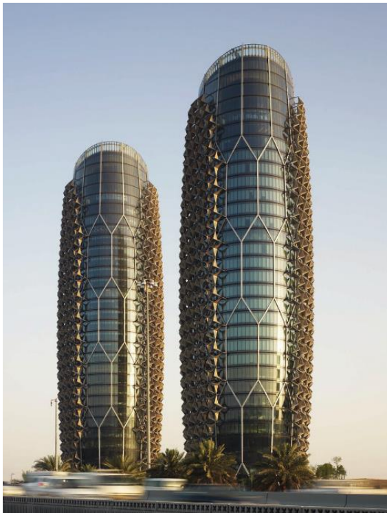
Figure 7 - 4: Modernized Mashrabiya shadings of Al-Bahr Towers, Abu Dhabi (Oborn, 2013)
