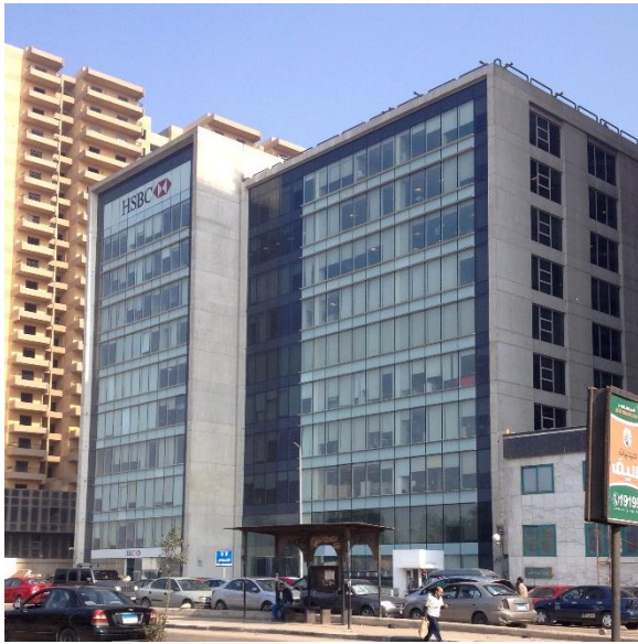
Figure 1 - 2: HSBC Bank, in Maadi district, Cairo. The fully glazed façade is facing the west orientation overlooking the Nile river. Disregarding the pleasant Nile view, the occupants pulled their internal opaque curtains, and turned electric lights on as a response for protection against the solar radiation (By researcher).
