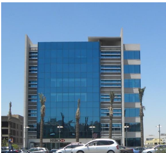
Figure 1 - 7: HSBC Bank, in the 5th settlement, Cairo. The building is a low-rise office building with highly glazed façade. The design exhibits the poor environmental and climatic considerations for hot-arid climates (By researcher).
