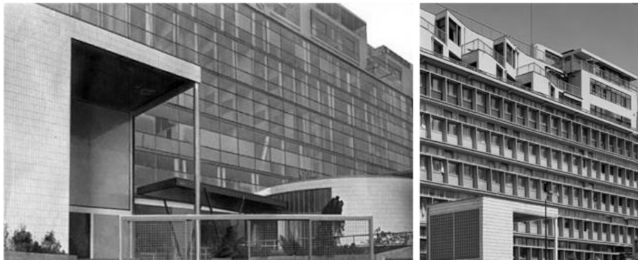
Figure 3 - 15: La Cite de Refuge, Paris, Le Corbusier, before and after adding solar protection (Butera, 2005)
