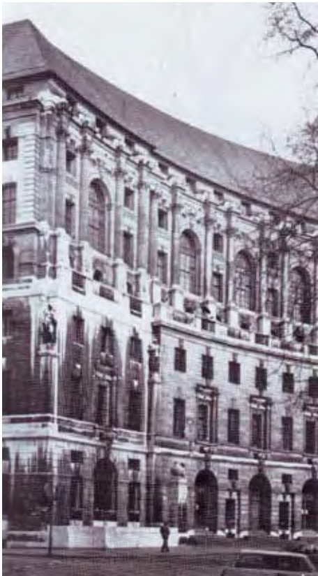
285. Sir Edwin Lutyens, Britannica House , London (1924-1927). Umbau durch Peter Inskip and Peter Jenkins Architects (1987-1989).
