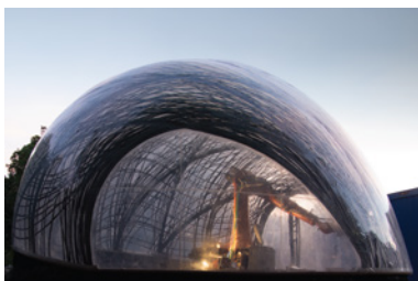
Fig. 4.4.18: The relation between the industrial robot and the composite shell; source: ICD/ITKE University of Stuttgart.
