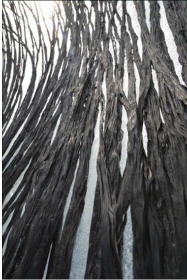
Fig. 6.4.4: The laid fibers on the formwork; source: ICD/ITKE University of Stuttgart.
