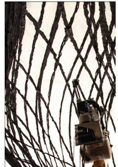
Fig. 4.4.20: The process of laying fibers on the membrane.
