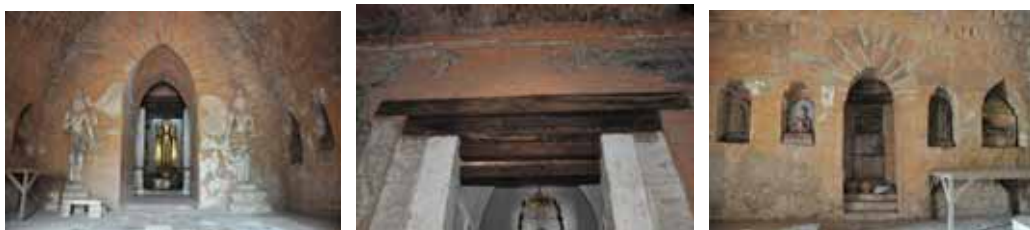
Fig 5.40: Timber members mixing with masonry elements and multilayer vaults using stone and bricks mixed in Naga-Yon temple
