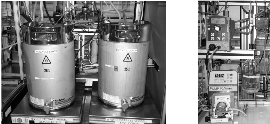
Figure 7.4 left: Substrate tanks on balances; right: dosing pumps.
