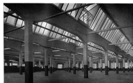
W 370 Shedhalle Bau D 1913 WAYSS & FREYTAG 1925
