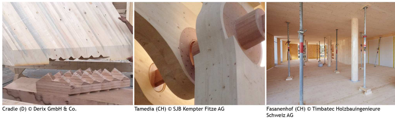
Figure 10. Details in T3: A glueless demountable LVL beech connection (left); a custom CNC oval beechwood pin connection (mid); new glued connections in the TS3 system (right).
