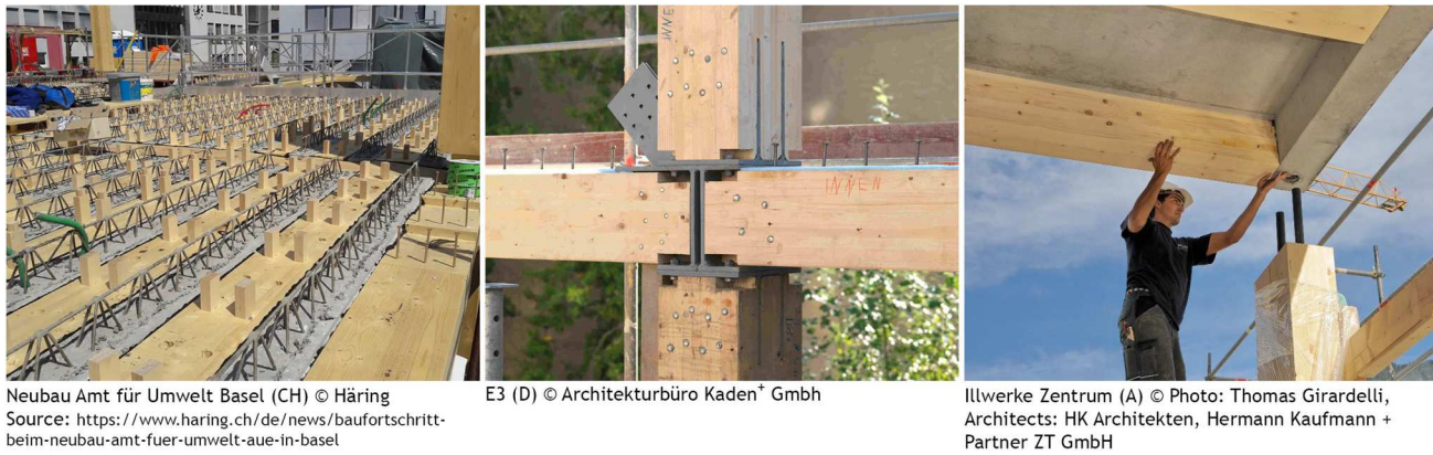
Figure 7. Variety of details in T2: Prefabricated wood and concrete elements with steel inlays prior to adding reinforcement, ductwork, and concrete on site (left); steel connection (mid); simple connection for assembly of the CREE ribbed ceiling system (right).
